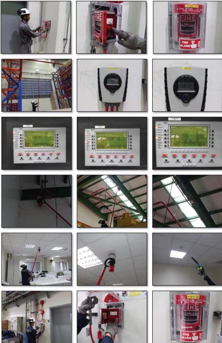
Picture of Testing Fire Alarm System (GC 19)
